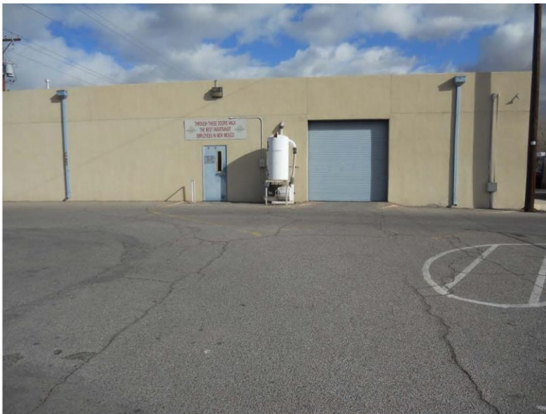
Figure – Building 2, West Elevation
